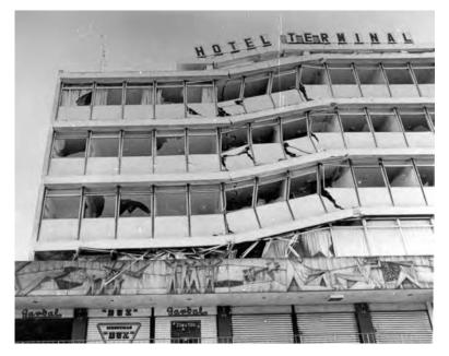
Figure 93 Guatemala earthquake 1976. Collapse of the Hotel Terminal in Guatemala City, caused by the failure of reinforced concrete columns in its third story. 1976.
