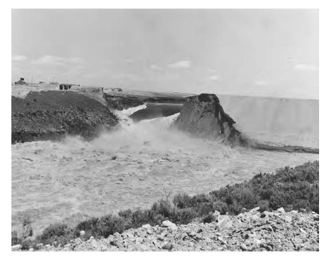
Figure 95 Failure of the Teton Dam.
