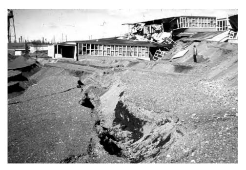
Figure 80 Alaska earthquake, March 27, 1964. Government Hill Elementary School in Anchorage which was destroyed by the Government Hill landslide.
