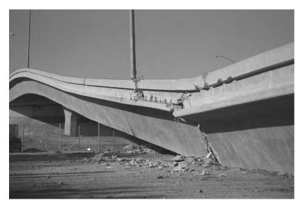
Figure 115 Road collapse caused by Northridge earthquake.
