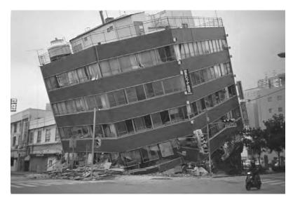
Figure 117 An office building with a partially destroyed first floor. The majority of partial or complete collapses were in the older, reinforced concrete buildings built before 1975.
