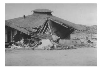
Figure 66 Collapsed school in Kern County, California, earthquake, 1952. The Cummings Valley School completely collapsed. The school building was reportedly constructed in 1910 of concrete walls and a wood roof. The building was a total loss.
