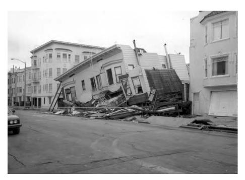
Figure 108 Loma Prieta, California, earthquake, October 17, 1989. Structures damaged in the Marina District of San Francisco. The first story of this three-story building was damaged because of liquefaction; the second story collapsed. What is seen is the third story.
