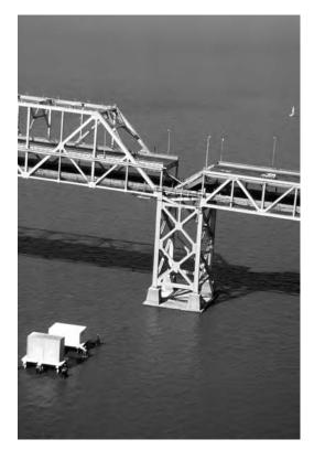
Figure 107 Loma Prieta, California, earthquake, October 17, 1989. Roadbed collapse near the interface of the cantilever and truss sections of the San Francisco–Oakland Bay Bridge.
